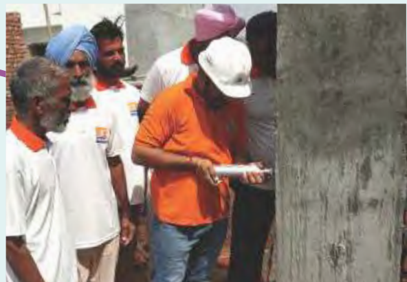
On site cement strength check
