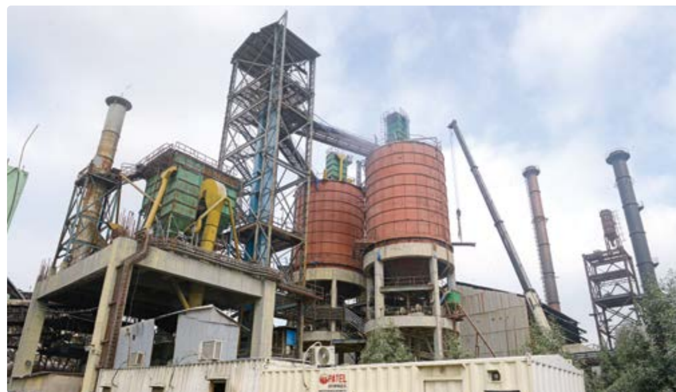
Synthetic Gypsum Plant at Ras
