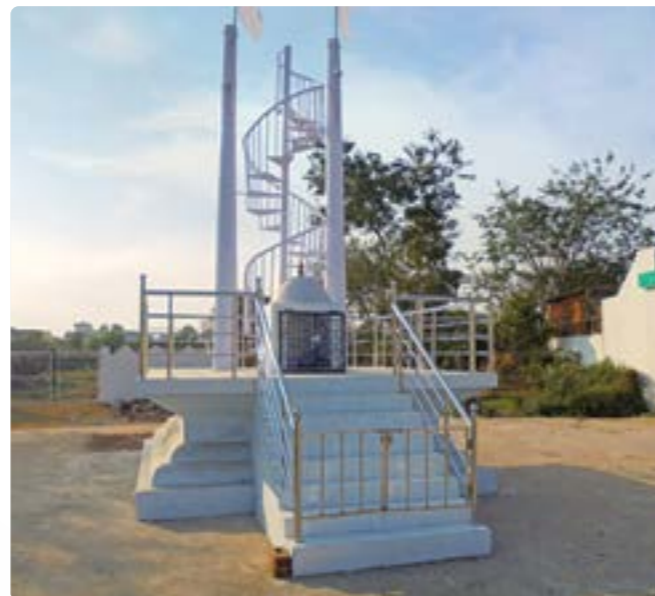
Construction of Jait Khamb for socio-cultural activities as part of CSR
