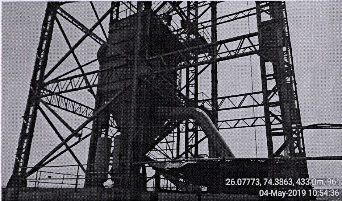
Dust collector at transferred Points.
