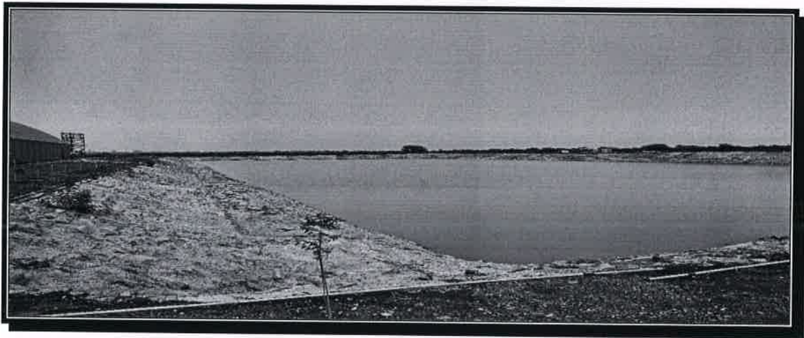
Rain Water Harvesting Pond Near Reclaiimer of 1 Lac KL Capacity.
