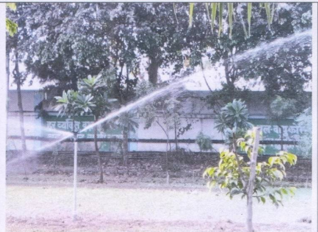
Installed Water Sprinkler System
