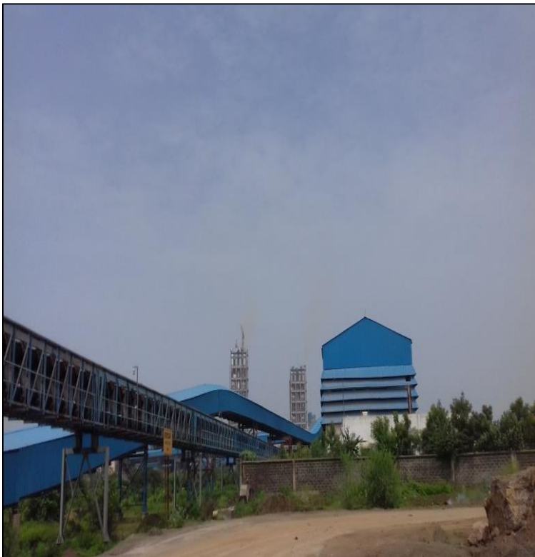
Photo no. 11 Showing covered conveyor
