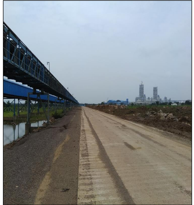
Photo no. 12-Showing cemented haul road
