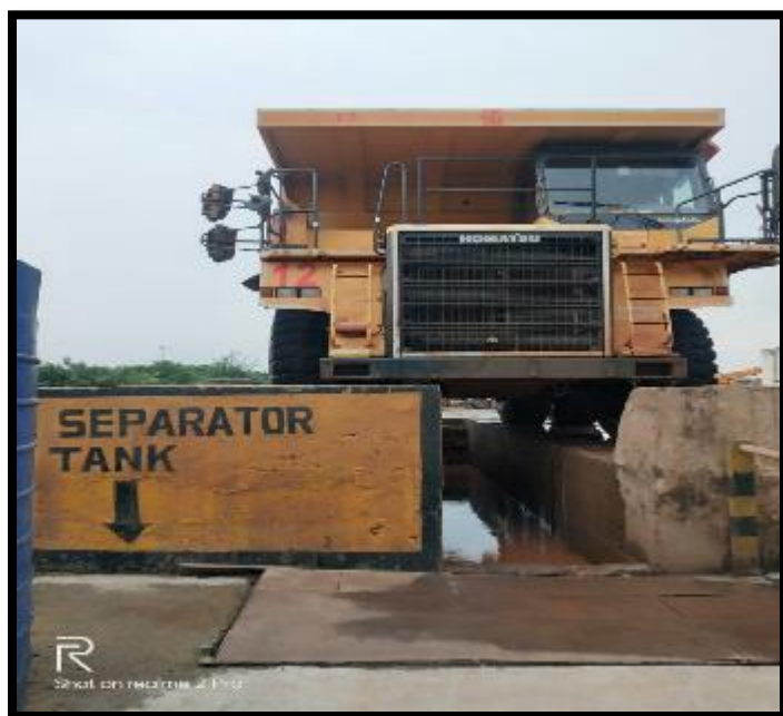
Photo 9: Showing Washing Ramp provided for servicing of HEMMS
