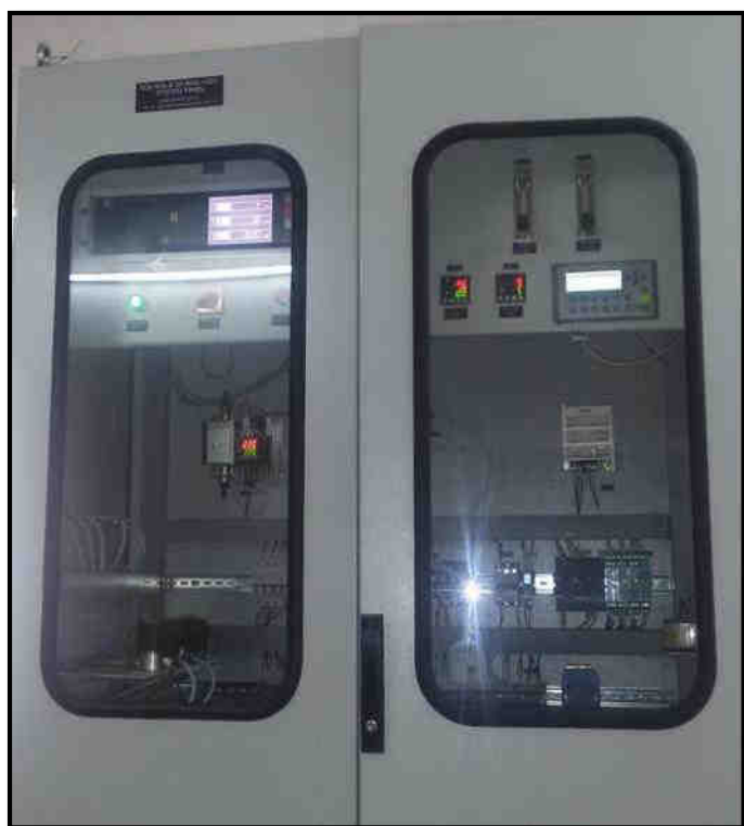
Photo no. 1 - Showing CEMS installed at Raw Mill Kiln Stack Unit-1
