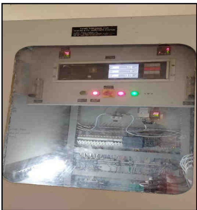
Photo no. 2 - Showing CEMS installed at Raw Mill Kiln Stack Unit-2
