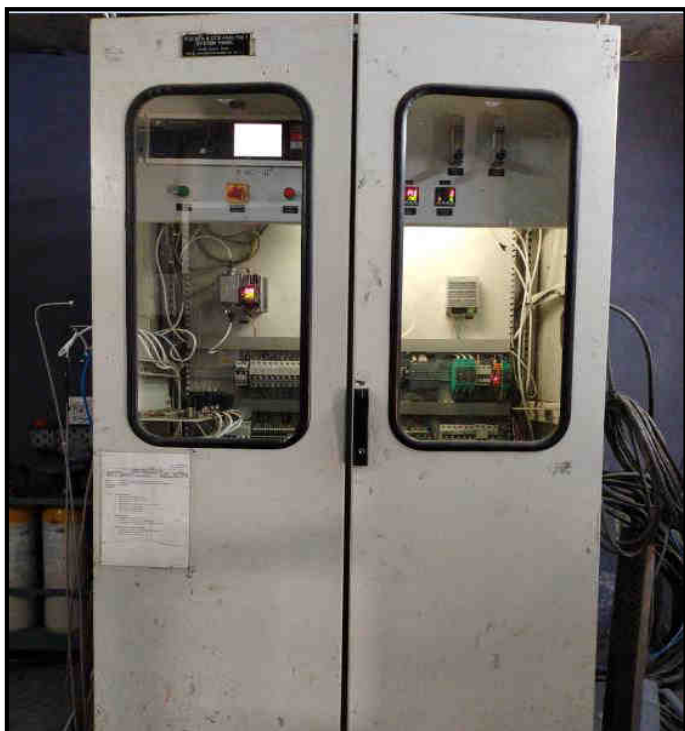
Photo no. 3 - Showing CEMS installed at Captive Power Plant
