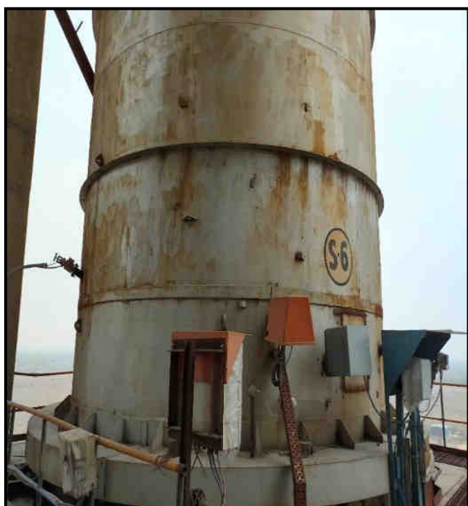
Photo no. 2 - Showing CEMS installed at Raw Mill Kiln Stack Unit-2
