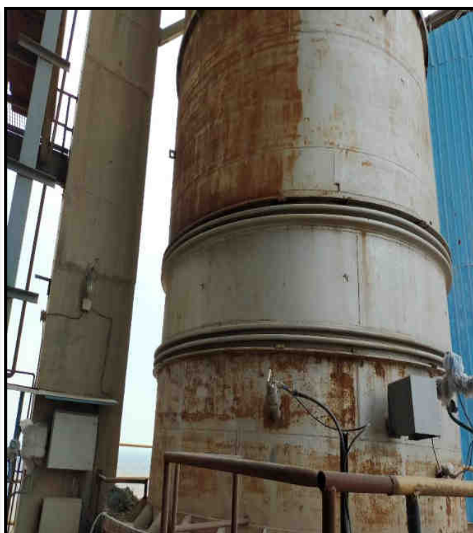
Photo no. 1 - Showing CEMS installed at Raw Mill Kiln Stack Unit-1
