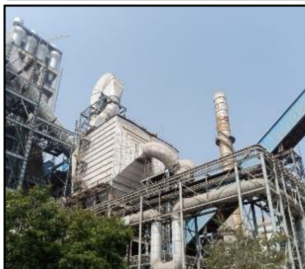
Photo 11: Showing Line-2 Cooler ESP
