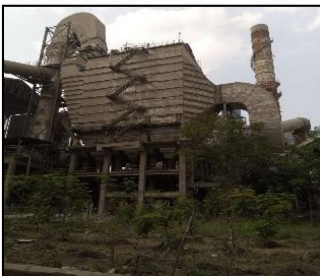
Photo 10: Showing Line-1 Cooler ESP
