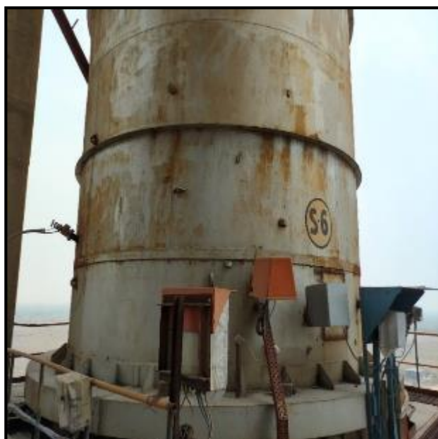
Photo 2: Showing CEMS installed at Raw Mill Kiln Stack Unit-1I
