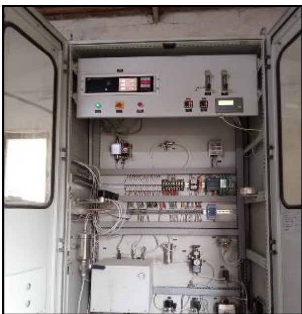
Photo 1: Showing CEMS installed at Raw Mill Kiln Stack Unit-1
