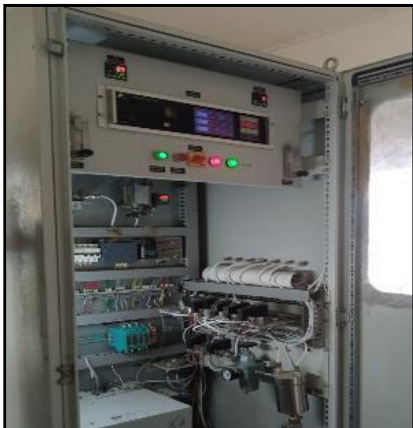
Photo 2: Showing CEMS installed at Raw Mill Kiln Stack Unit-1I
