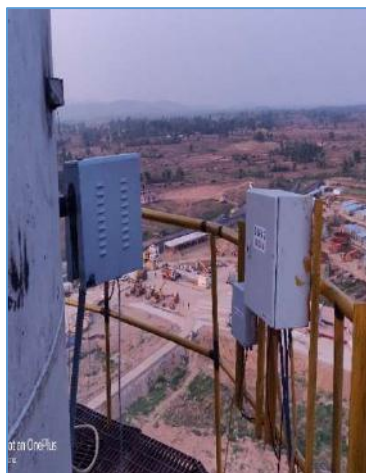
Opacity meter installed at Cement Mill Stack
