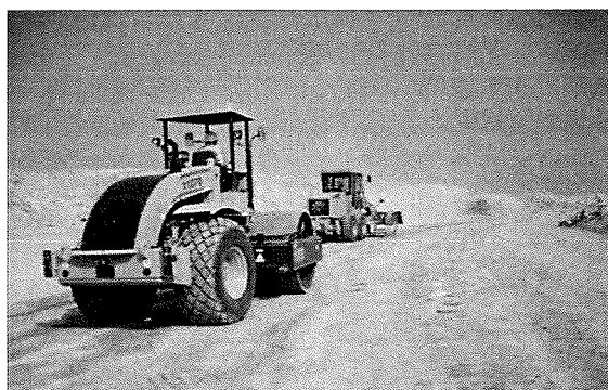
Haul Road with water spray compaction, grading
