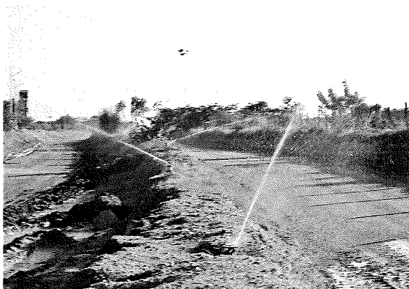
Haul Road with water spray compaction, grading
