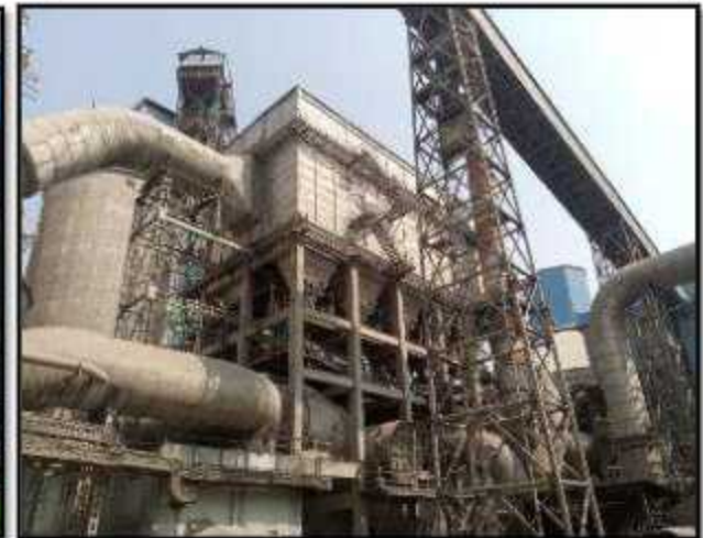
Photo 8: Showing Line-2 Cooler ESP
