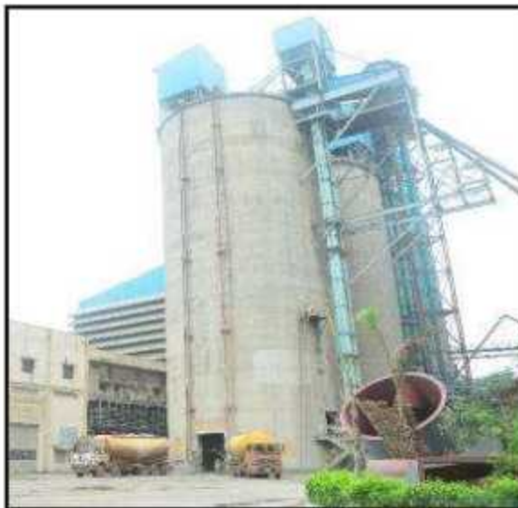
Photo 16: Showing fly ash Silo
