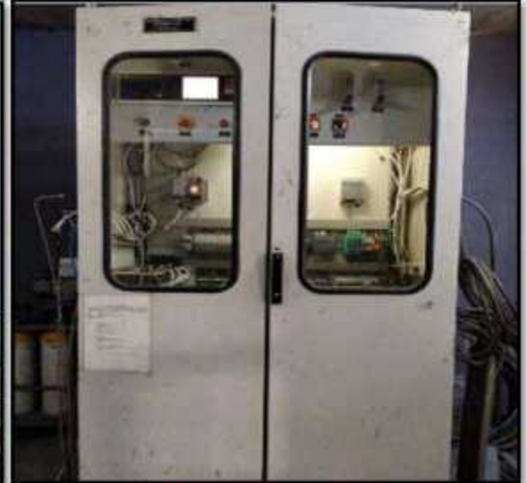
Photos showing CEMS installation
