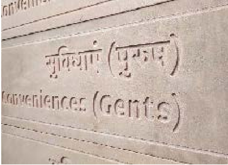
Dry Stone Panel ready for Epoxy
