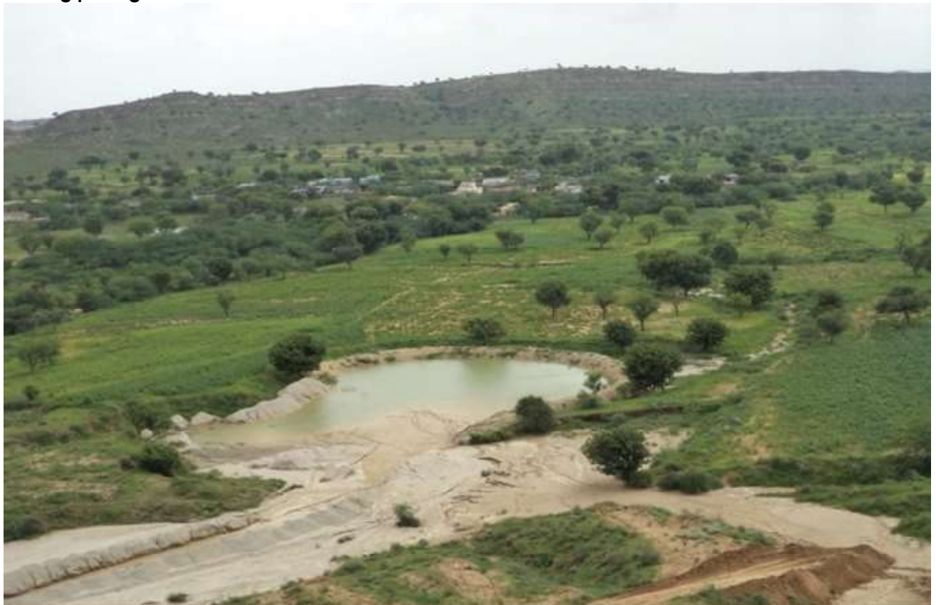
Desilting pit at garland drain
