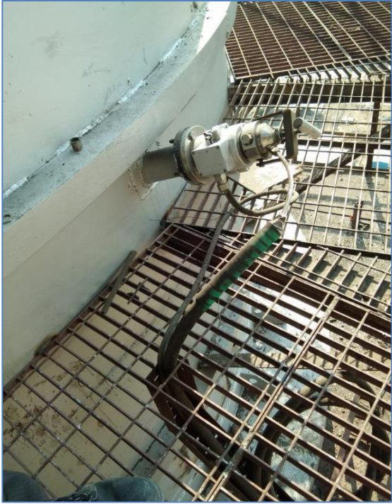
Gas- CEMS analyser installed at Raw/ kiln stack
