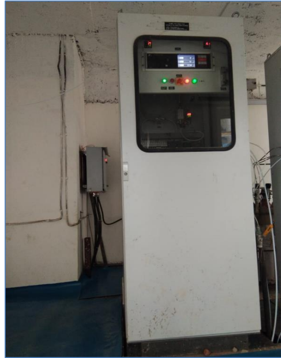
Gas- CEMS analyser installed at Raw/ kiln stack
